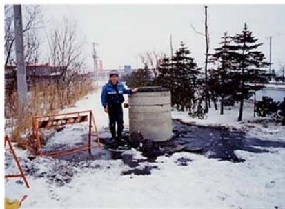
Photo 3. Uplifted sewer manhole in Kushiro Town. Photo 4. Investigation work.
